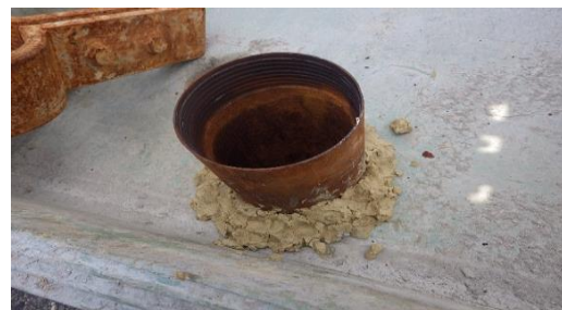
写真-6 遮水状況-2
