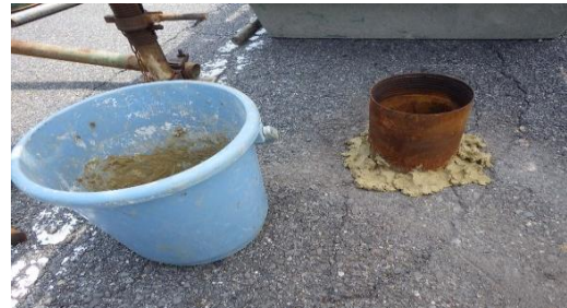
写真-5 遮水状況-1
